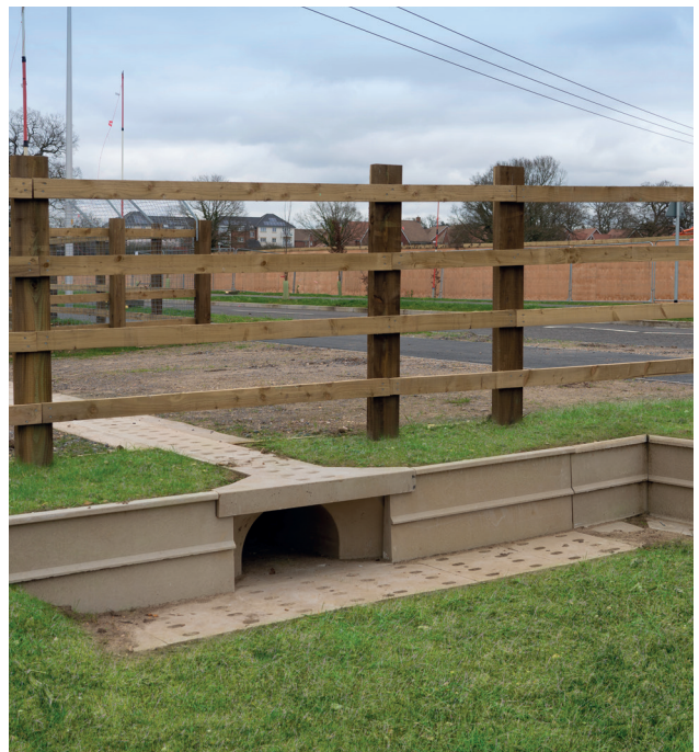
Ashridge Farm using tunnels to connect green infrastructure
