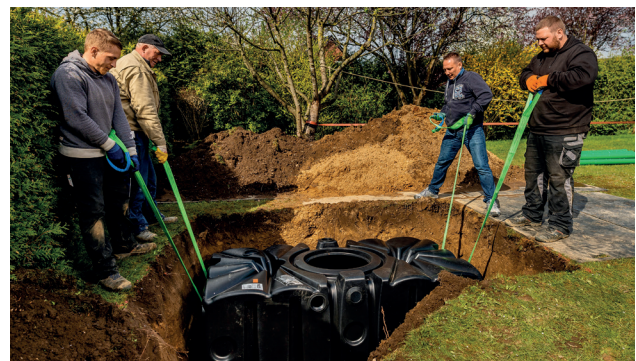
Installation of a Rainwater Harvesting Tank
